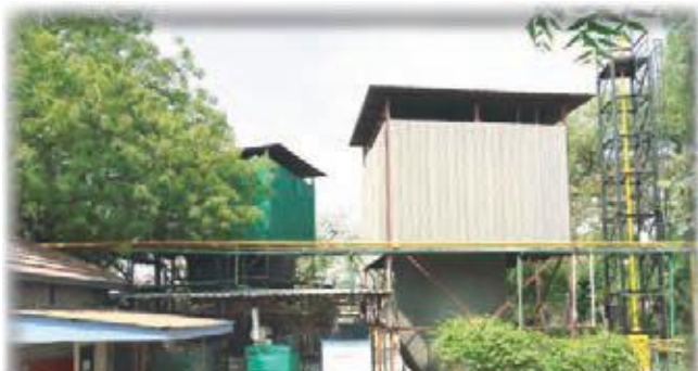
Bio Gas plant at MIL unit-1
