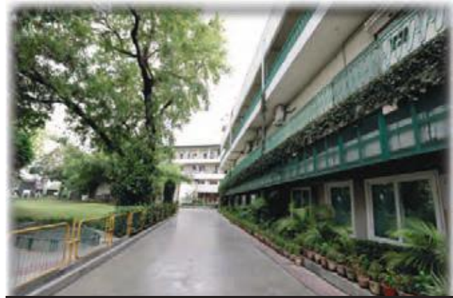
Administrative Bock at MIL plant, Hapur
